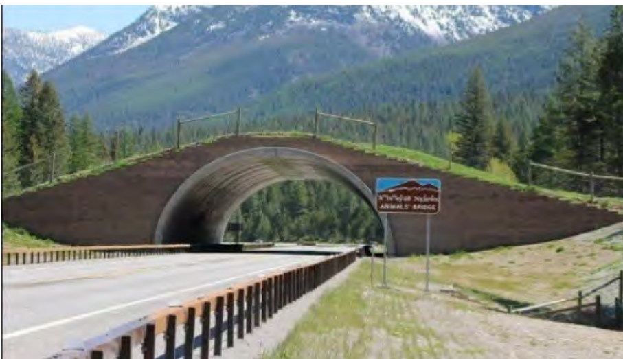
Examples of an animal-only crossing structure (left) and vehicle bridge modified with extensive plantings to promote wildlife movement (right).
